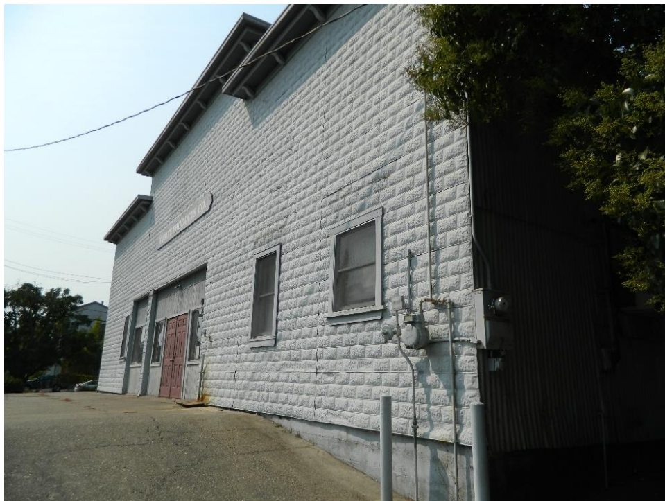
Figure 14. Photograph showing the primary façade, facing west.
