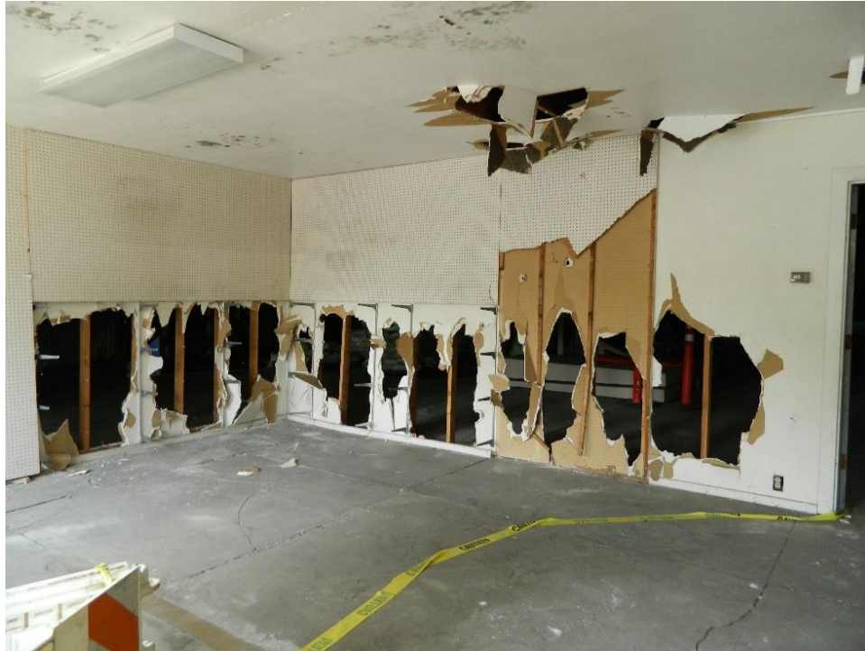
Figure 21. Photograph showing the interior "lobby" portion of the building.
