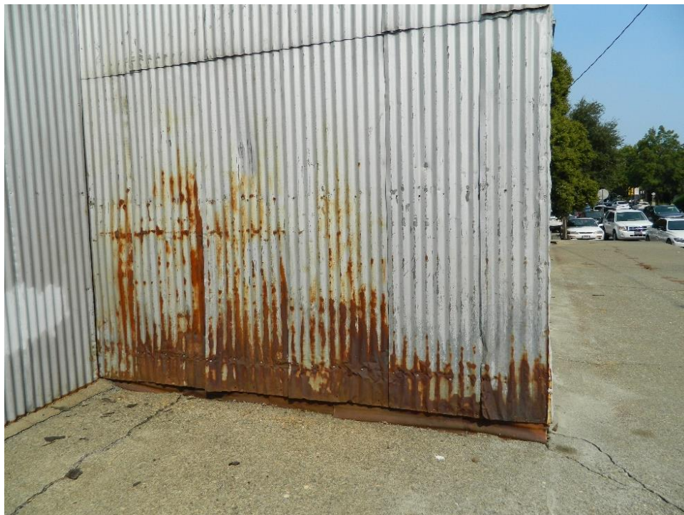
Figure 17. Photograph showing the west elevation shed addition, facing south.
