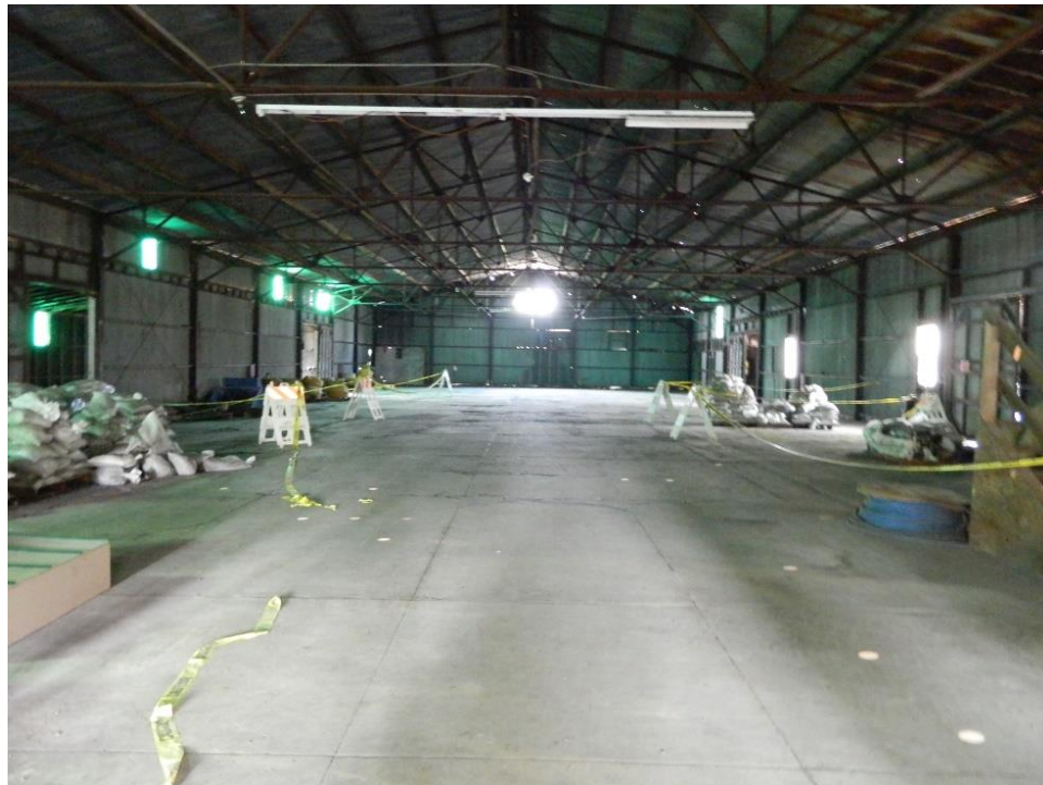
Figure 22. Photograph showing the interior of the building, facing north.
