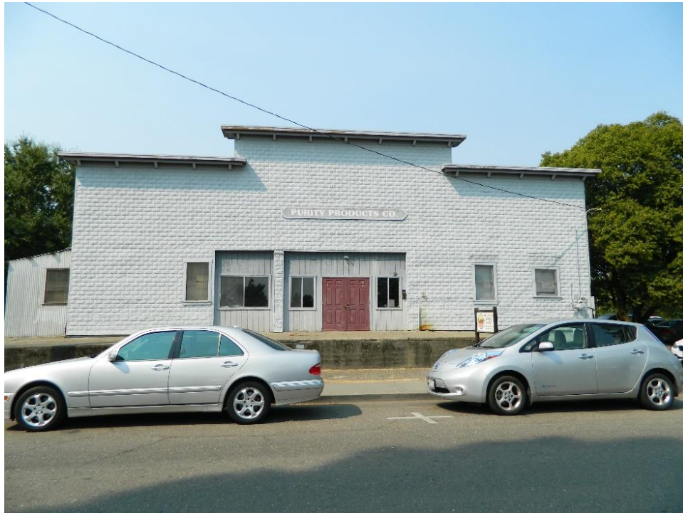
Figure 13. Photograph showing the primary façade, facing north.
