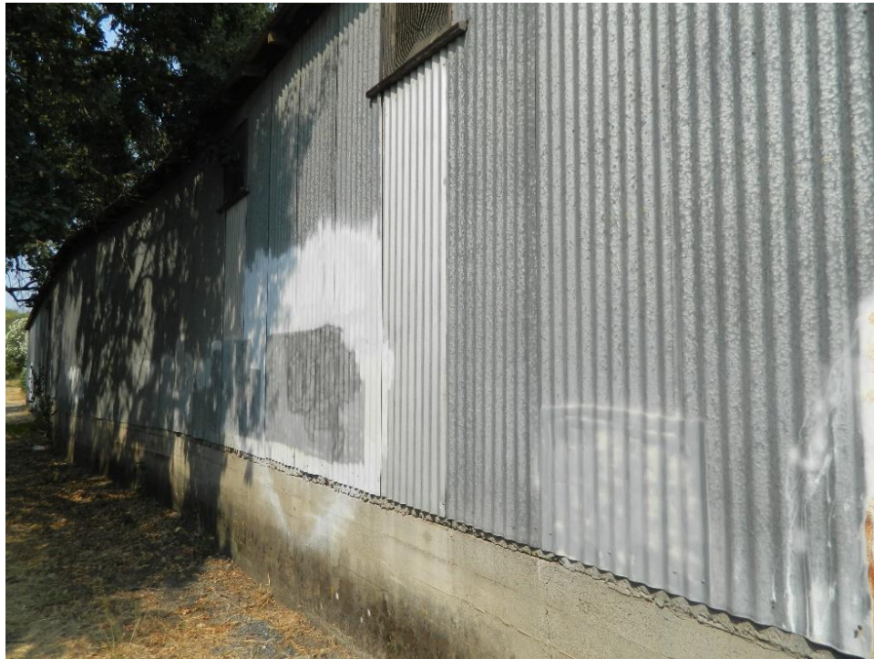
Figure 16. Photograph showing the west elevation, facing north.
