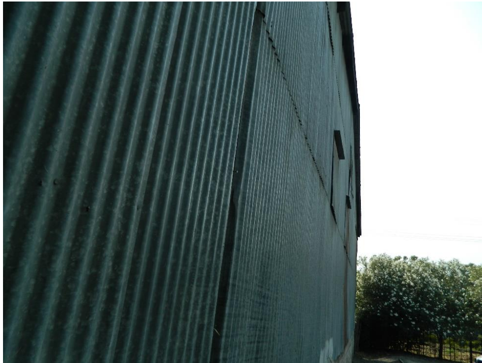
Figure 20. Photograph showing the north elevation, facing west.
